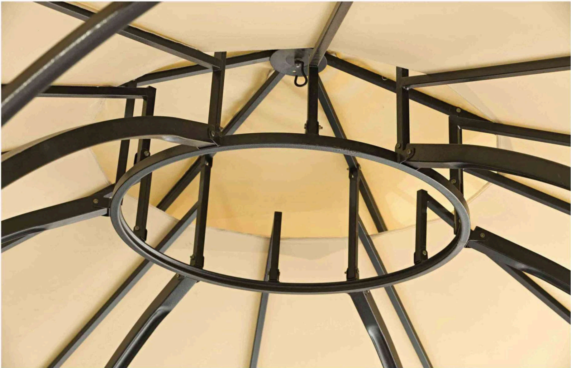
Reinforcement ring fixed in the shed
